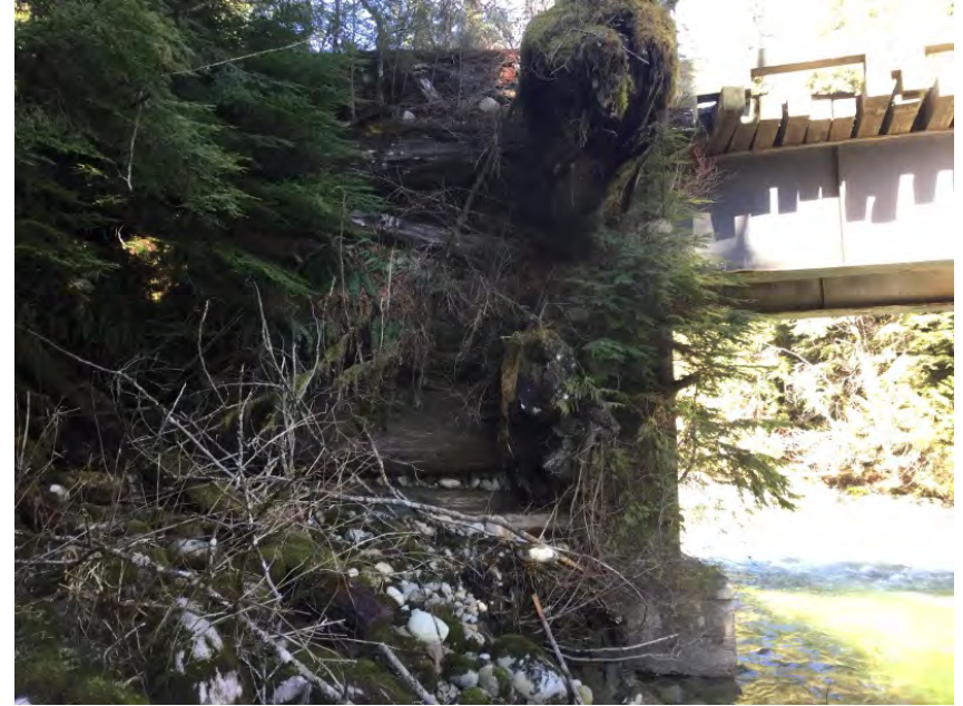
Downstream right bank condition
