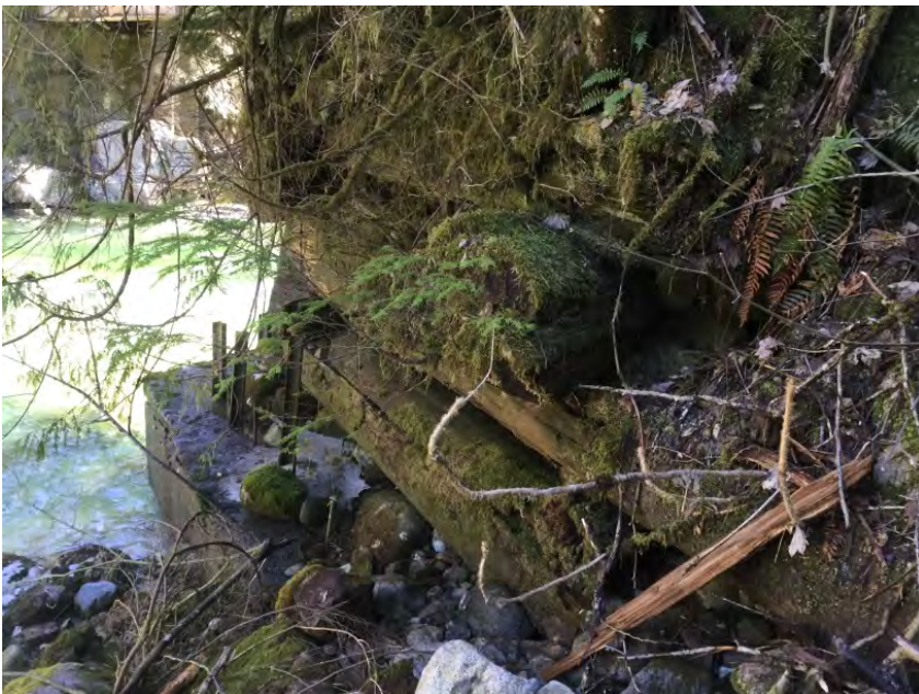
Upstream right bank wingwall condition
