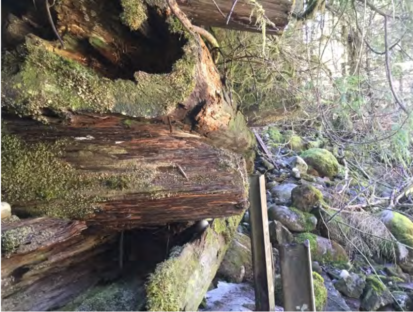
Upstream right bank wingwall condition
