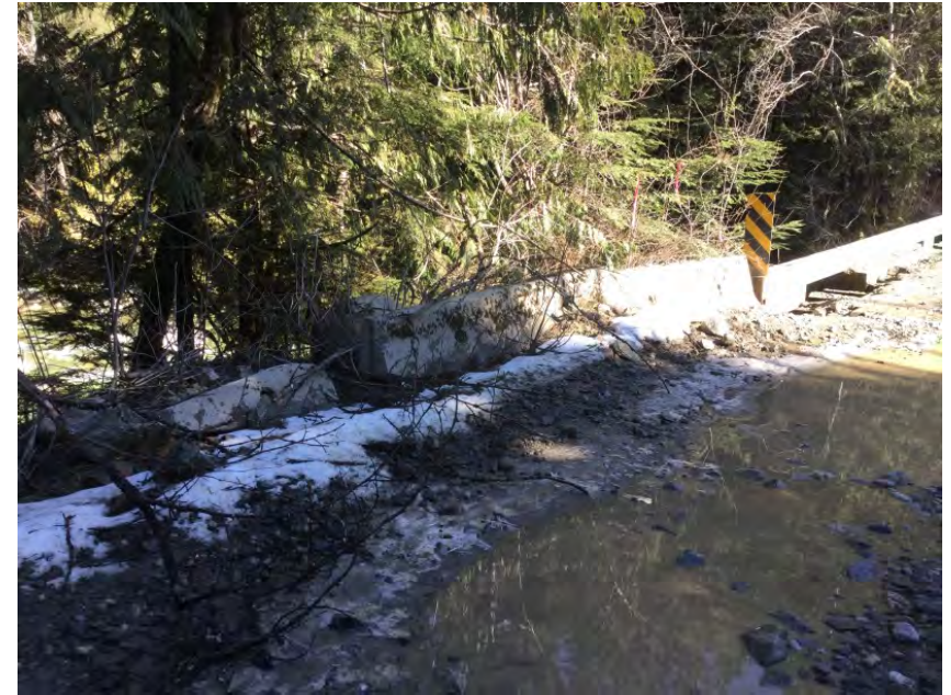
Upstream right approach no posts
