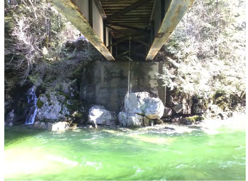
Left Bank Abutment when facing downstream
