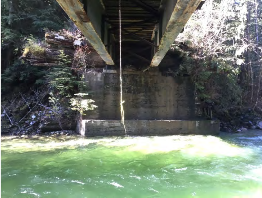
Right Bank Abutment when facing downstream
